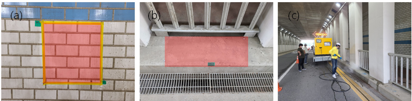
Figure 1. The surface area of roadway underpass structure for dust cleaning between (a) tile wall; (b) concrete pad foundation; (c) pressurized water jet cleaning.
