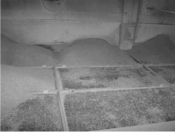
Figure 7. An accumulation of fly ash on SCR catalyst modules.
