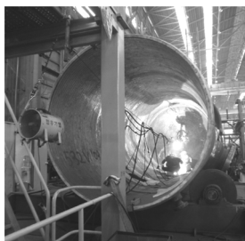
(a) Tunnel type of limited space
