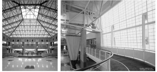
Figure 12. Two examples of translucent aerogel insulation as a high performance thermal insulation solution for daylighting[12].
