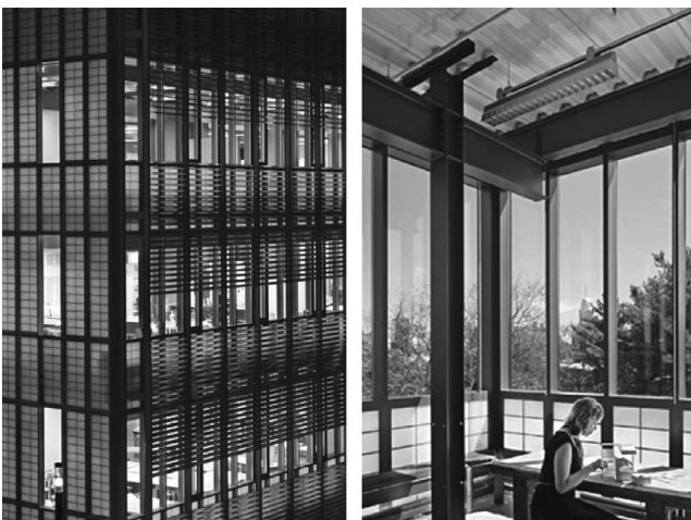
Figure 11. Translucent aerogel insulation used in a curtain wall at the sculpture building and gallery of Yale University[12].
